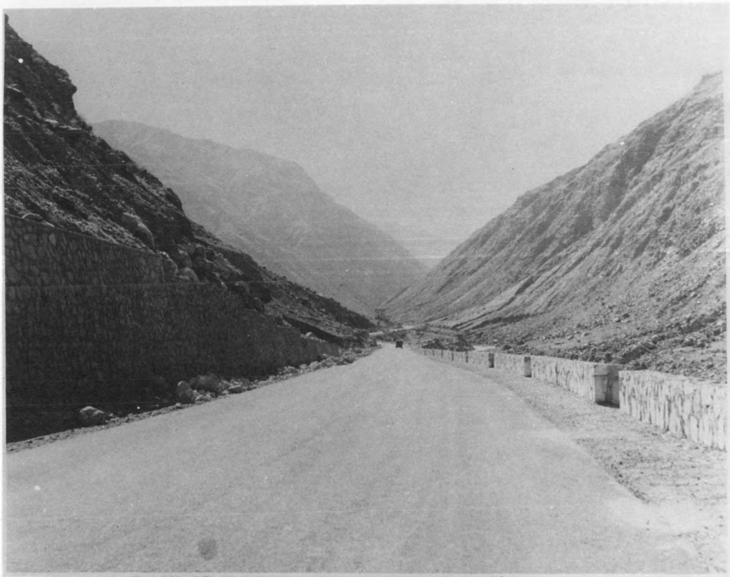
Plate 2 Retaining walls of this kind greatly increase the cost of road construction.
