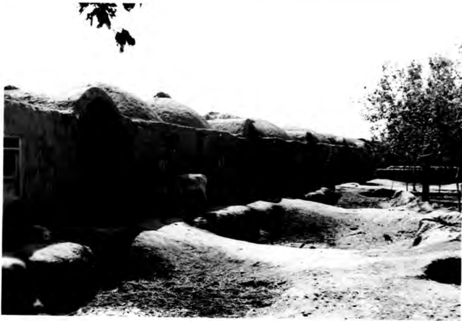
A further slight variation in house styles, showing barrel vaulted openings acting as porches each for two houses, one opening off either side.
