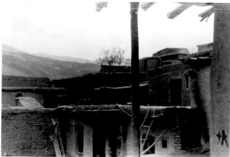
Close-up view of the structure of houses in Khanrud. The greater use of sun-dried brick is obvious as well as the abundance of wood in the structure.
