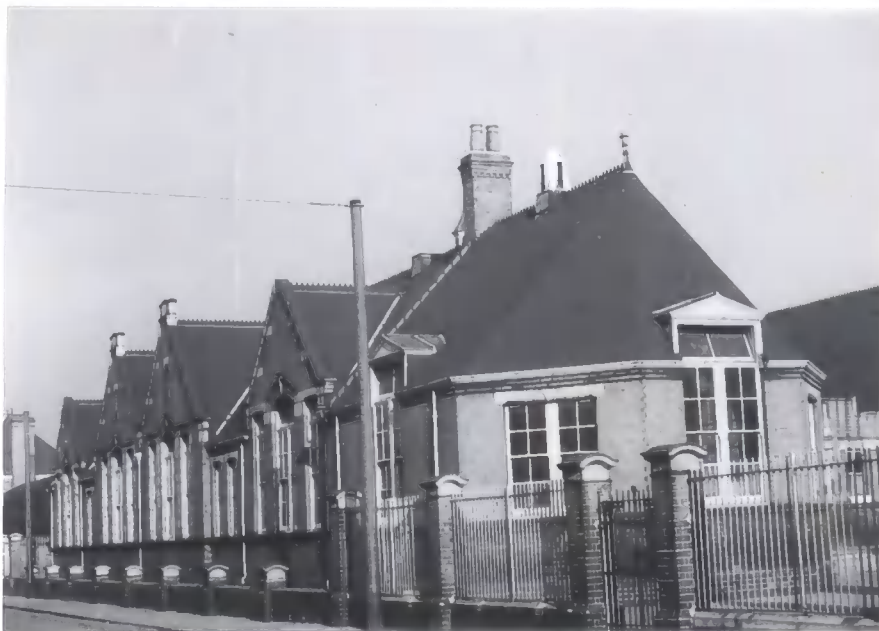
The Infant School built at Grangetown 1906. It also contained a cookery centre attended by girls from nearby schools.
