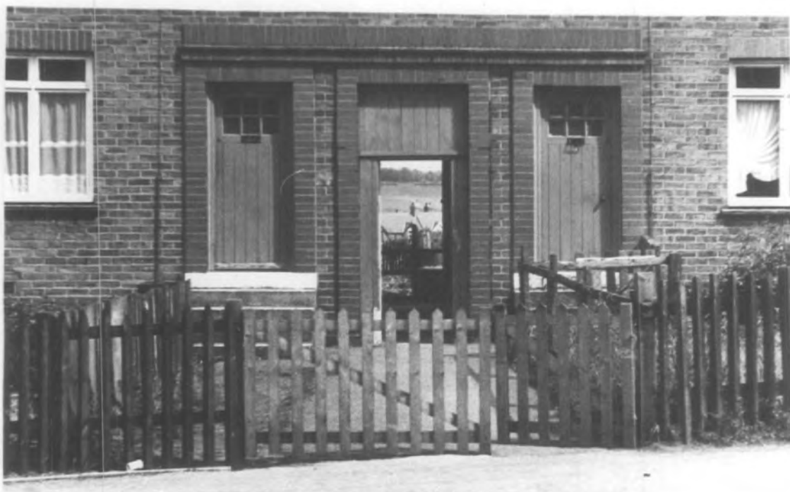
ILLUSTRATION 4-3 Pringle Place, New Brancepeth. A through-passage was the standard Tudor Walters method of improving rear access to blocks of four or more houses.
