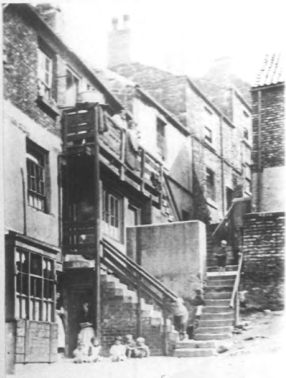
ILLUSTRATION 2-4 Bankwell Stairs, Pipewellgate, in the 1920s
