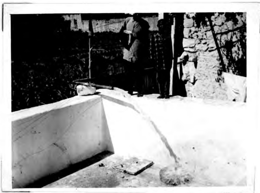
Plate 19(a) - A well with an electric pump, the water flows into a storage tank (jabia).
