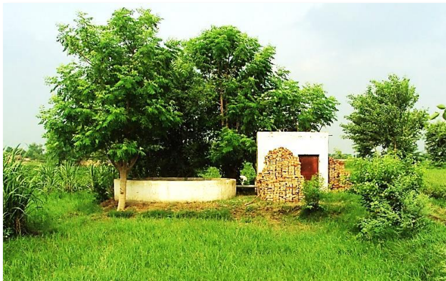
Picture 7.9: Sewerage Sump
