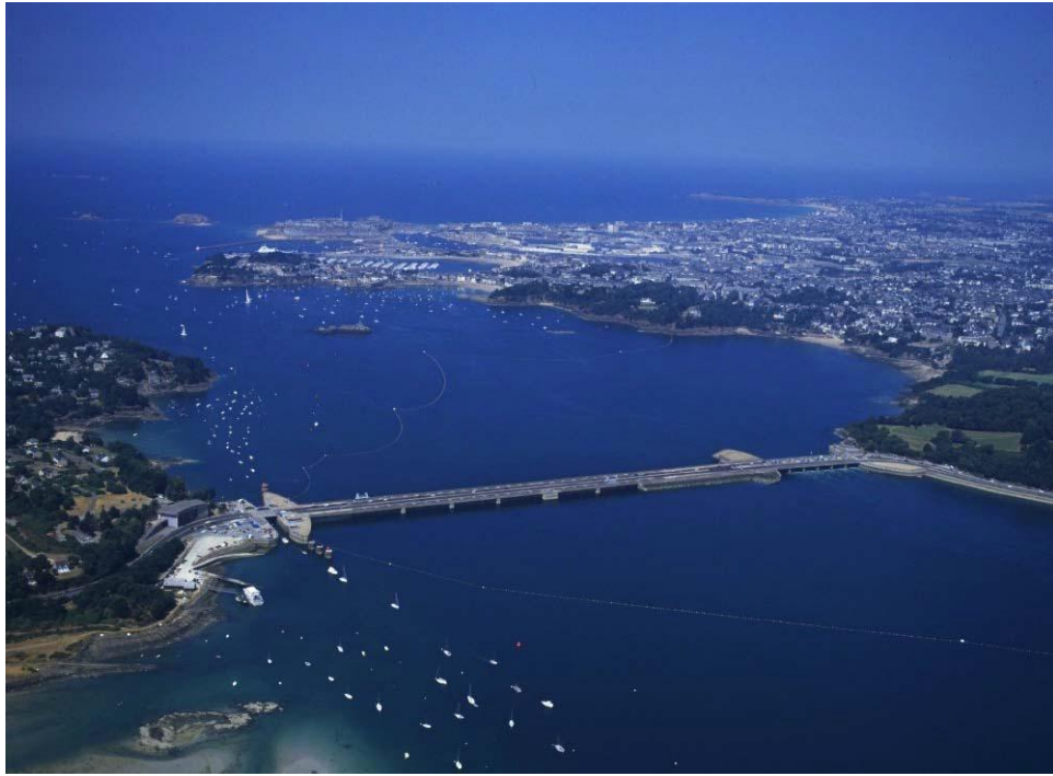
Figure 2.1 Tidal power plant, barrage type, at La Rance, France
