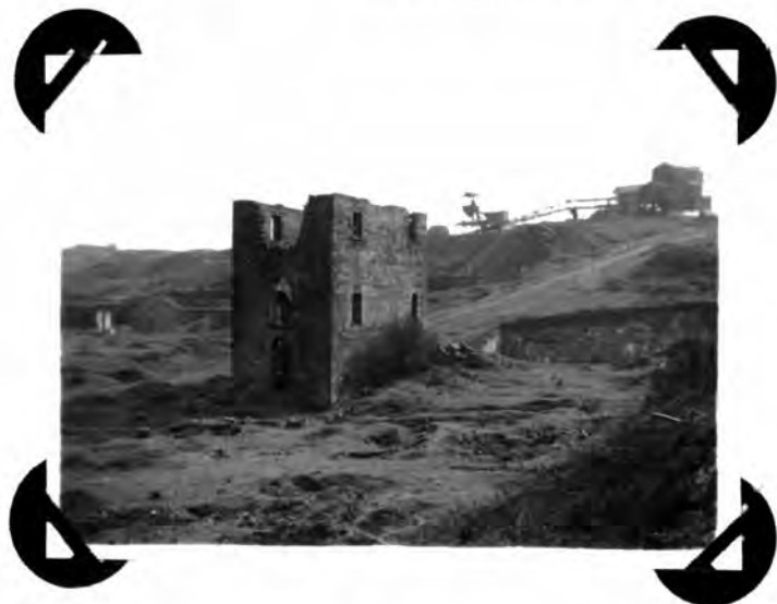
Engine House of Disused Iron Works.
