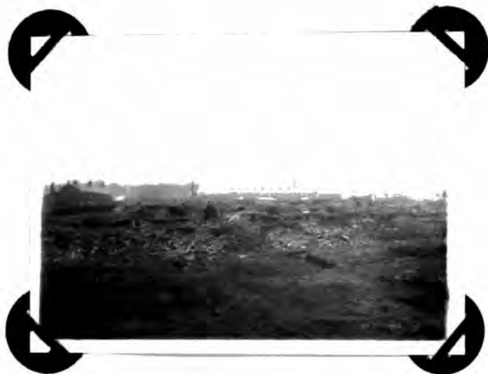
Derelict coke ovens and pit heaps at Low Beechburn Colliery.
