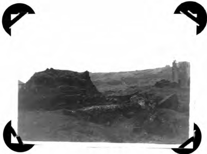
Iron and Slag core of blast furnace.
