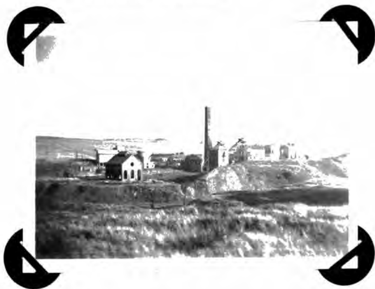
Derelict Colliery premises surrounded by colliery waste heaps. N.B. Newness of Washery plant on the left.
