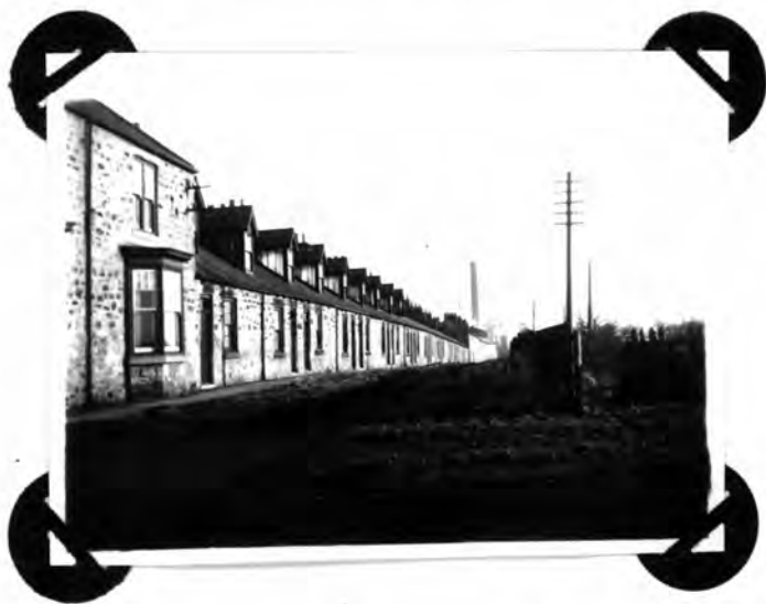
Thomas Street, Auckland Park with Colliery in background. N.B. Bend in roof-line at extreme end - due to subsidence.
