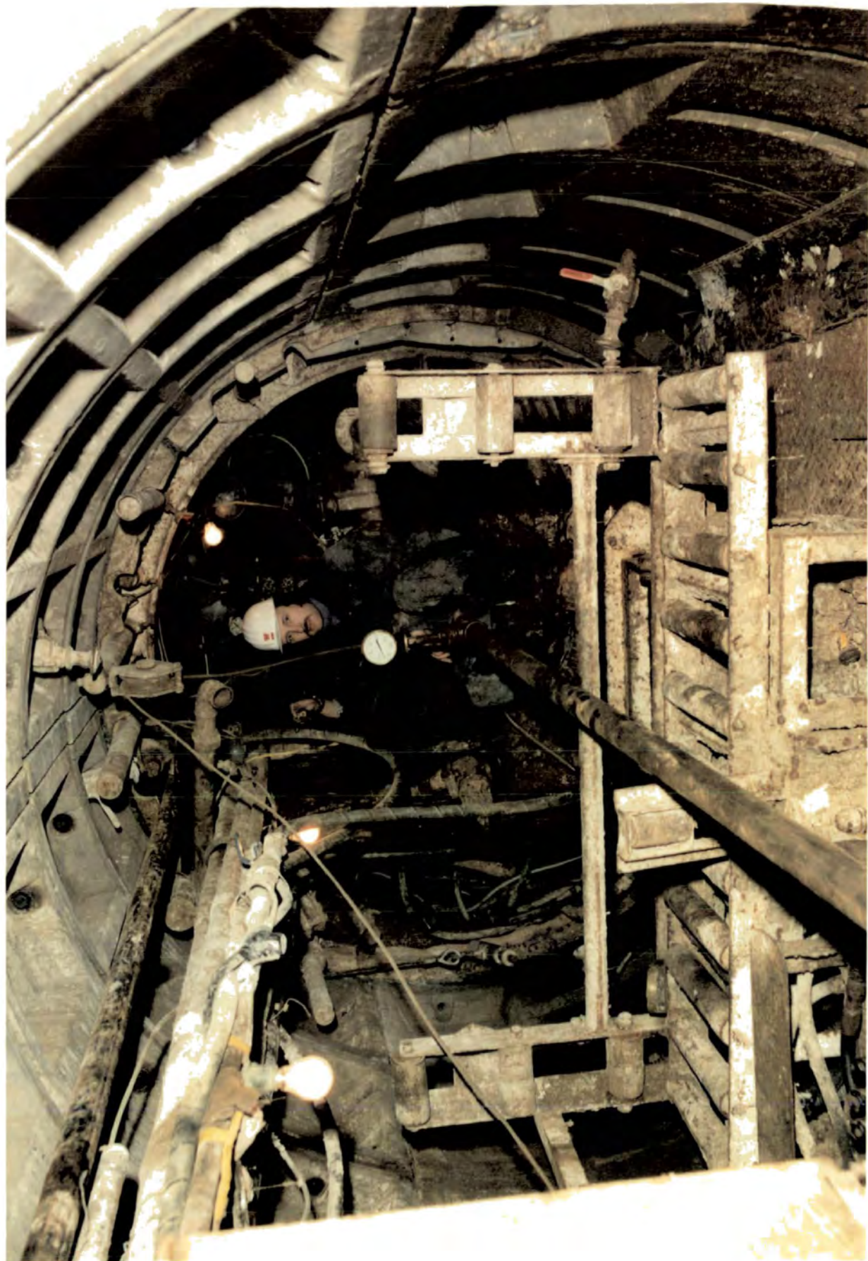
Plate 2.2 THE BENTONITE TUNNELLING MACHINE
