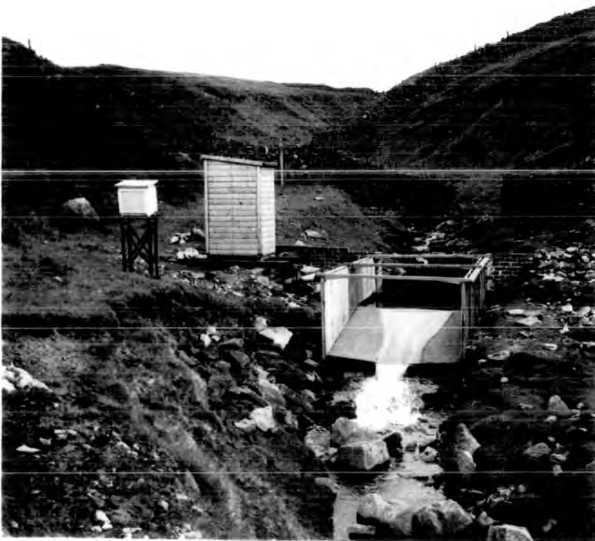
B COMPLETED WEIR
