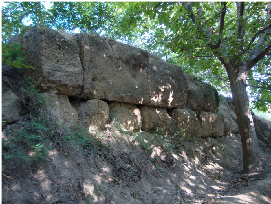
FIGURE 3-40: POSSIBLE FLOOD DEFENCES AT CARCHEMISH, JULY 2010 44
