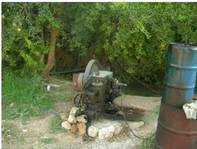
FIGURE 3-18: IRRIGATION PUMP ON THE RIVER SAJUR, JULY 2010 25
