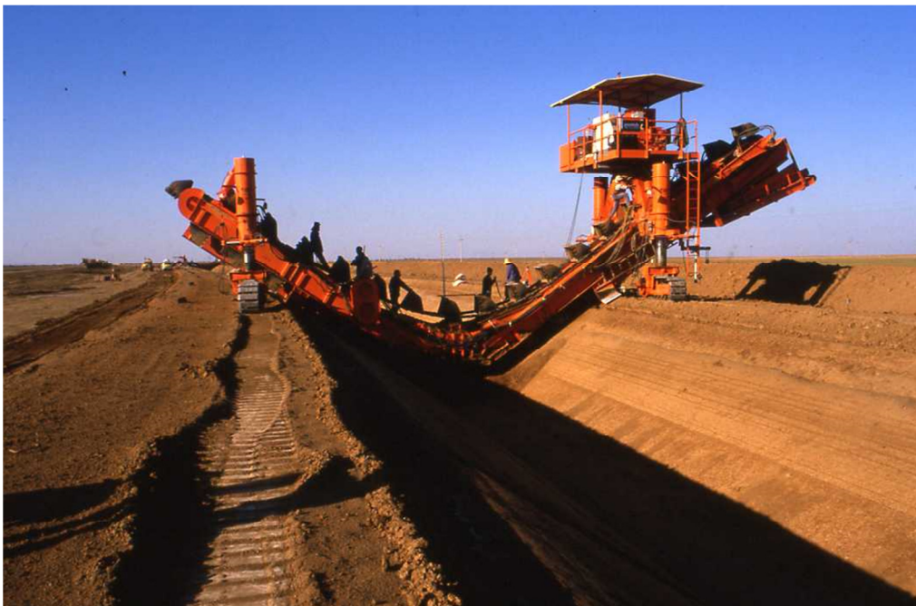
FIGURE 3-19: DIGGING OF A MAJOR IRRIGATION CHANNEL, IRAQ JAZIRAH 1985 26
