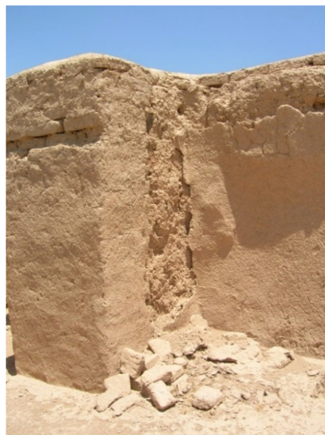
FIGURE 3-60: DEGRADED MUDBRICK WALLS AT TELL BRAK
