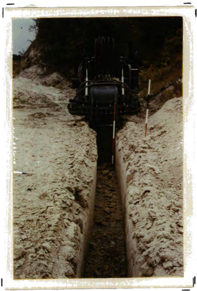
Plate 7.2 COMPLETED TRENCH , EXCAVATED ACROSS THE TUNNEL LINE .
