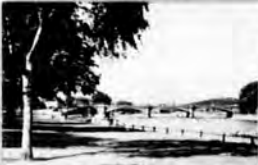
Tram Bridge from Victoria Embankment
