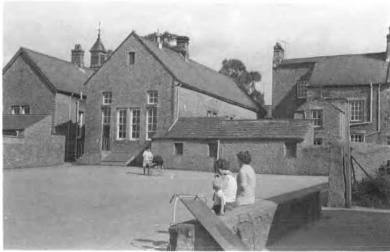
a. The original buildings
