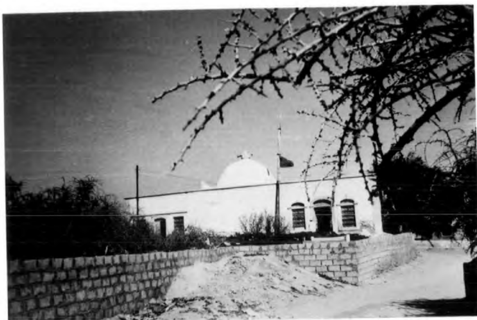
The Zāwiyah of Misurata as it looks from the North. On the right is the entrance of the Rawḍah , while the left entrance leads to the mosque behind it.
