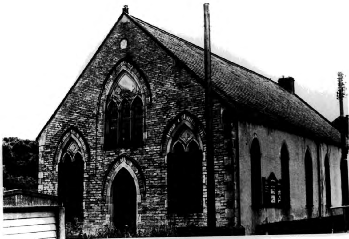
PLATE 9: a. Top ST. PAULS CHURCH, WATERHOUSES (1983) b. Bottom WESLEYAN METHODIST CHURCH, WATERHOUSES (1983)
