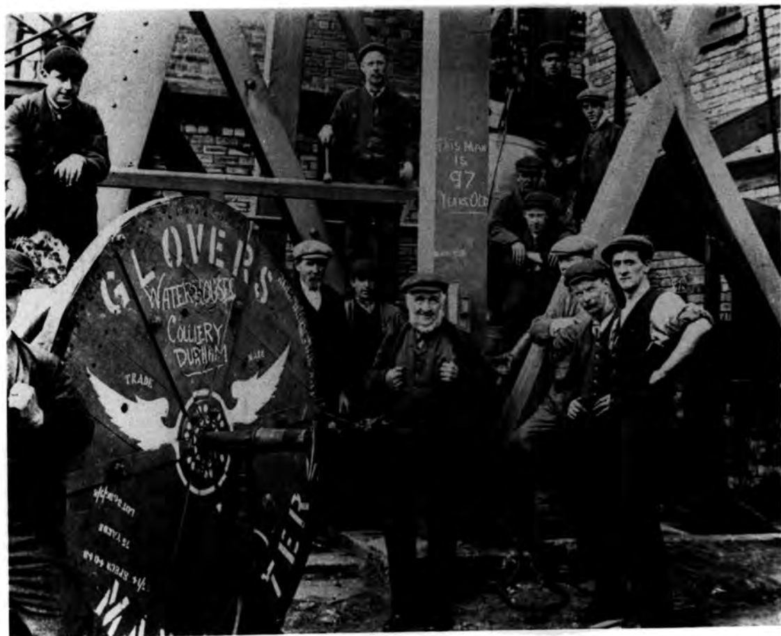
PLATE 17: a. Top SINKING A SHAFT AT ESH WINNING (undated) b. Bottom MEN AT THE WATERHOUSES UPCAST SHAFT (undated)
