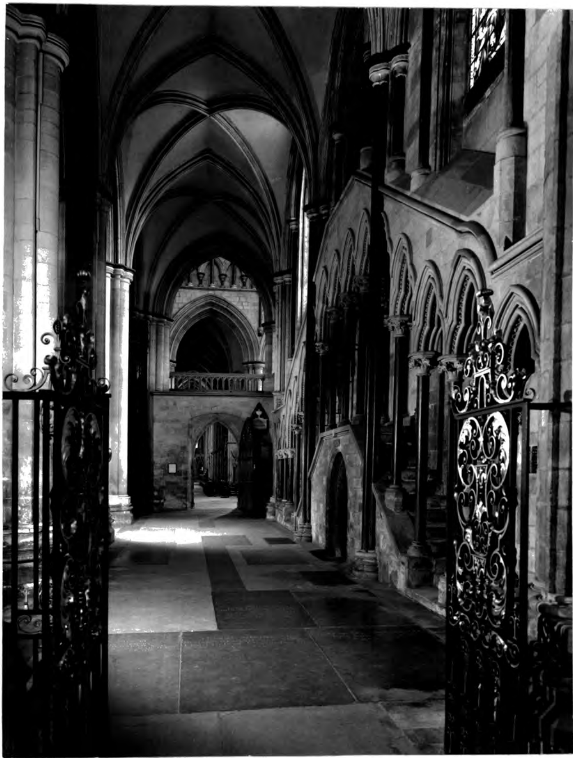
THE STAIRCASE TO THE CHAPTER HOUSE ENTRANCE
