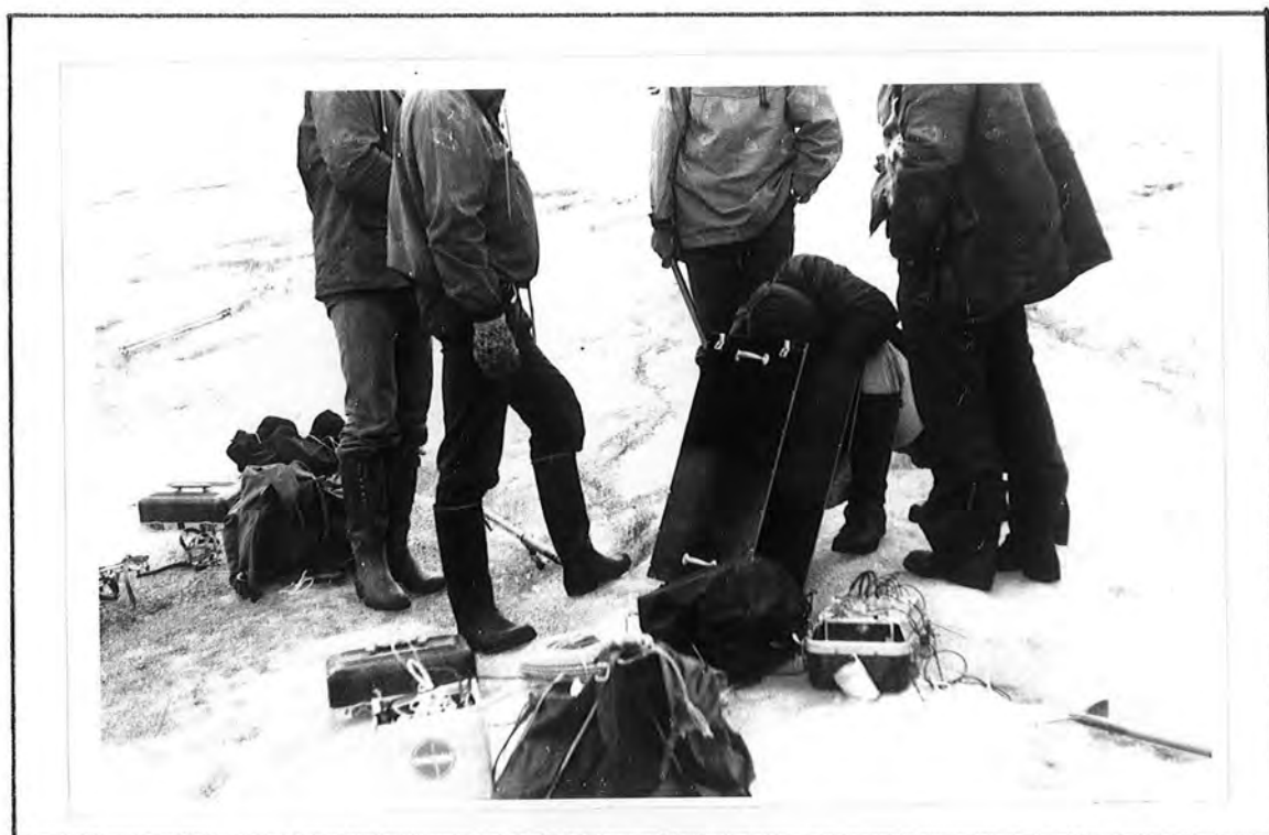
FIGURE 5.2 Setting up the Radio Echo-Sounding Equipment on Gljúfurárfjökull with Members of the Science Institute (University of Iceland).
