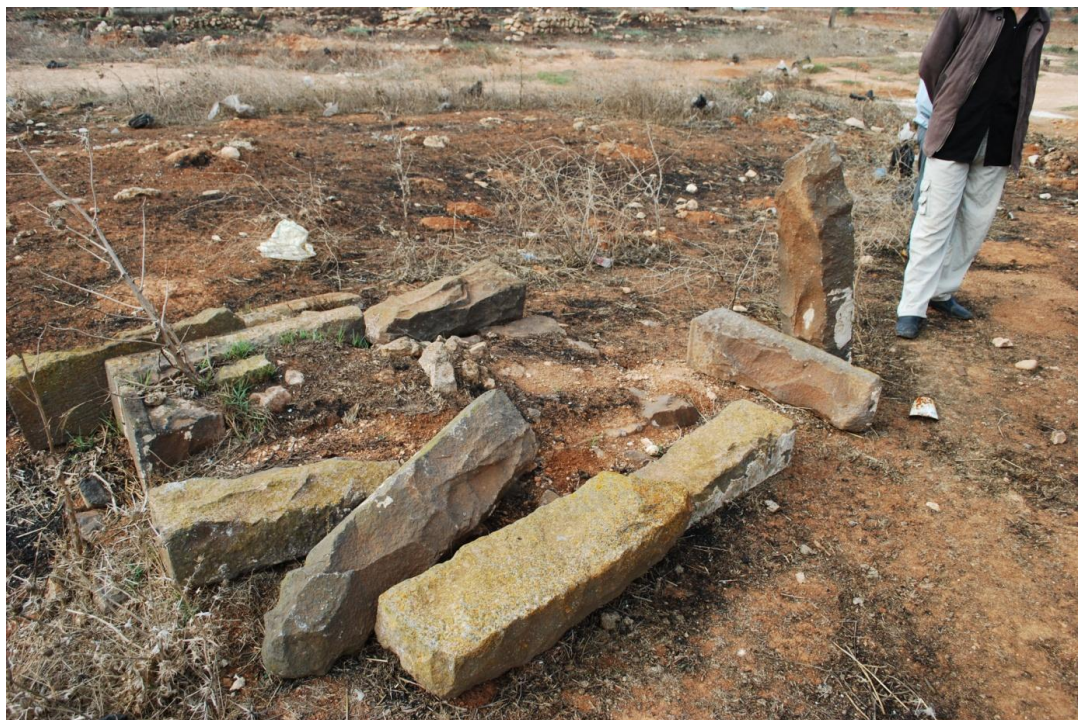
Figure 4.2. Image of re-use of earlier building lintels as grave revetments in an Islamic grave, Dmeini al Gharbiya, Homs Region (image courtesy of Dr Stephen McPhilips)
