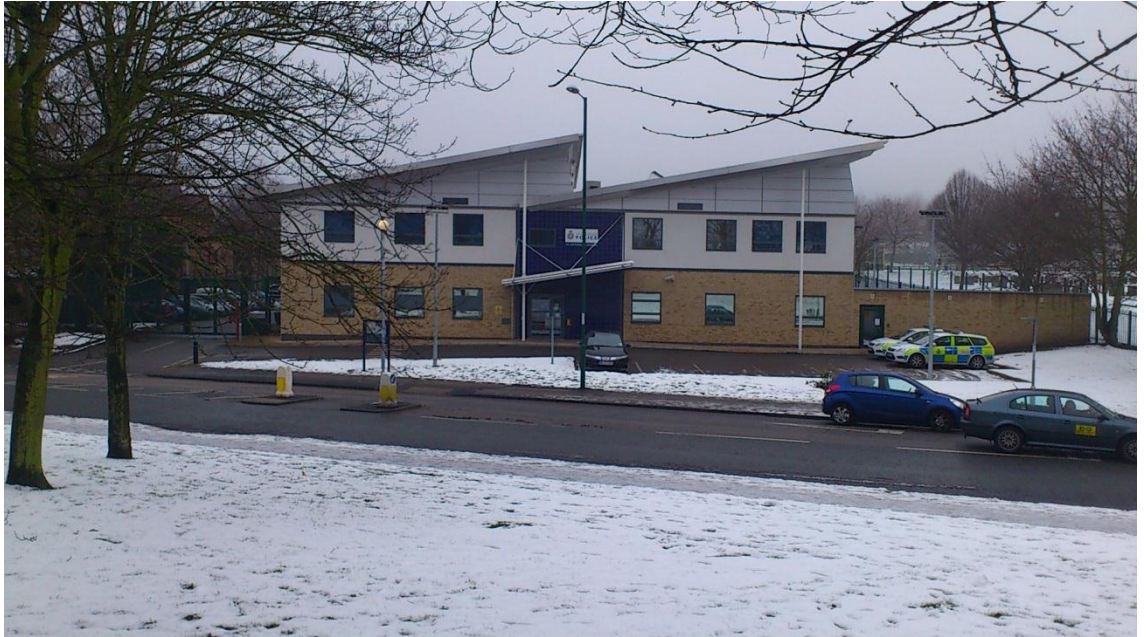
St. Ann's Police Station, St. Ann's, Nottingham: Photograph taken February 2012
