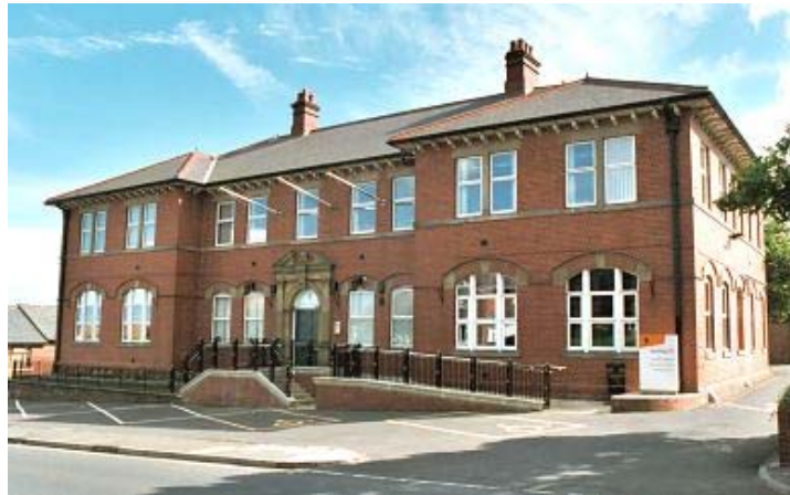
Figure 6.12: Building Ten: EDC ‘Main Building’
