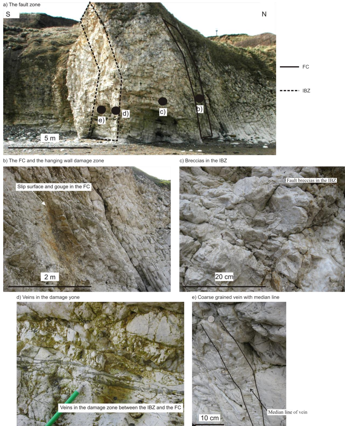
Figure 3.8 - Large displacement normal faults at Selwick Bay – outcrop scale
