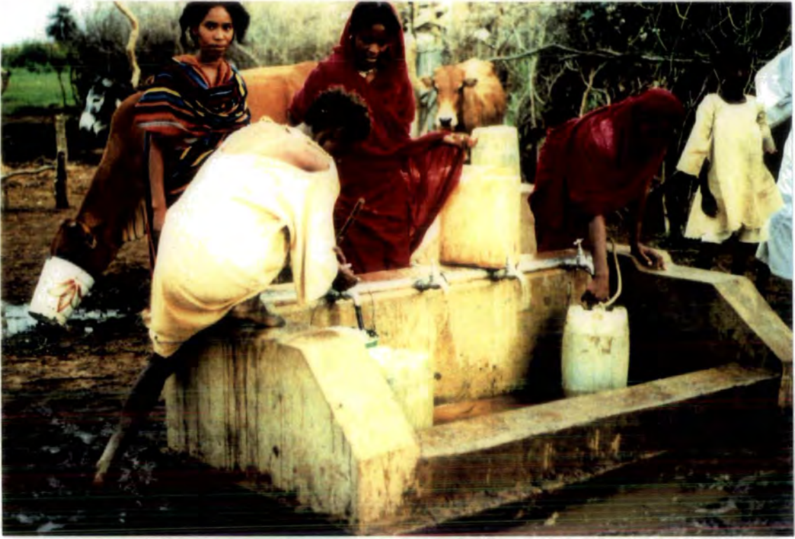
Plate 10: At Khammas Hajar wateryard several tapstands were damaged and the area surrounding the tapstands was very muddy.
