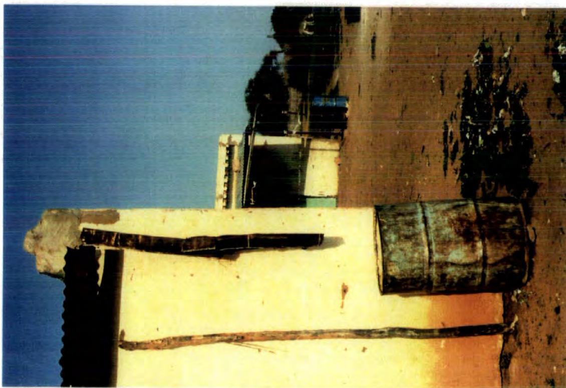
Plate 28: A sabaloka at the suq at Khammas Halab allows collection of rainwater from one of the relatively few metal roofs: a smaller-scale cistern.
