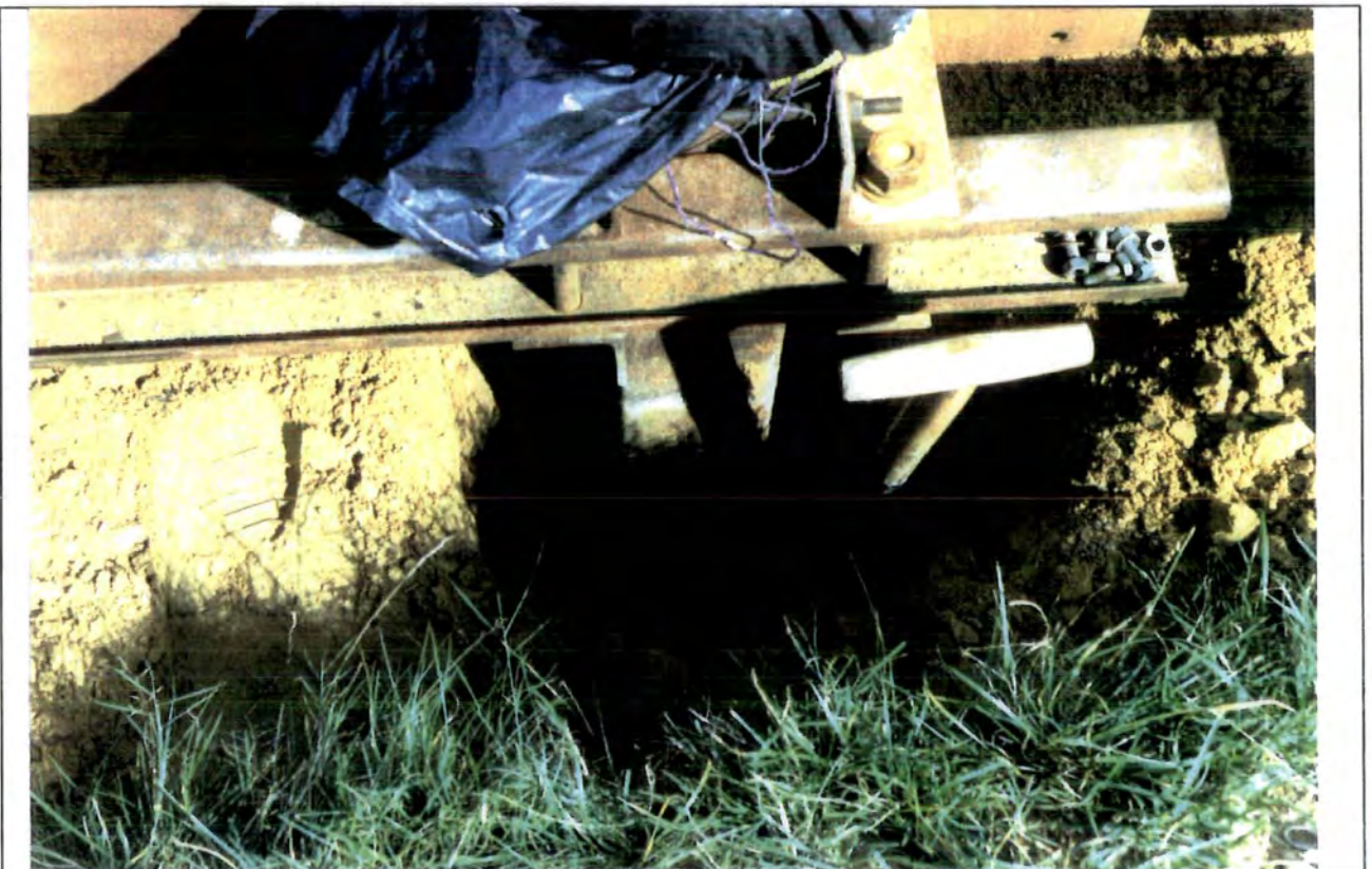
Plate 3.6 Excavation of sand around a pile.
