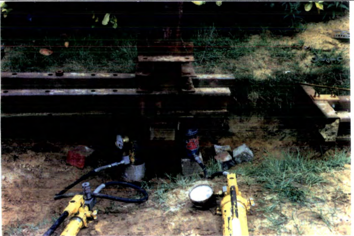
Plate 3.8 Pile extraction technique.
