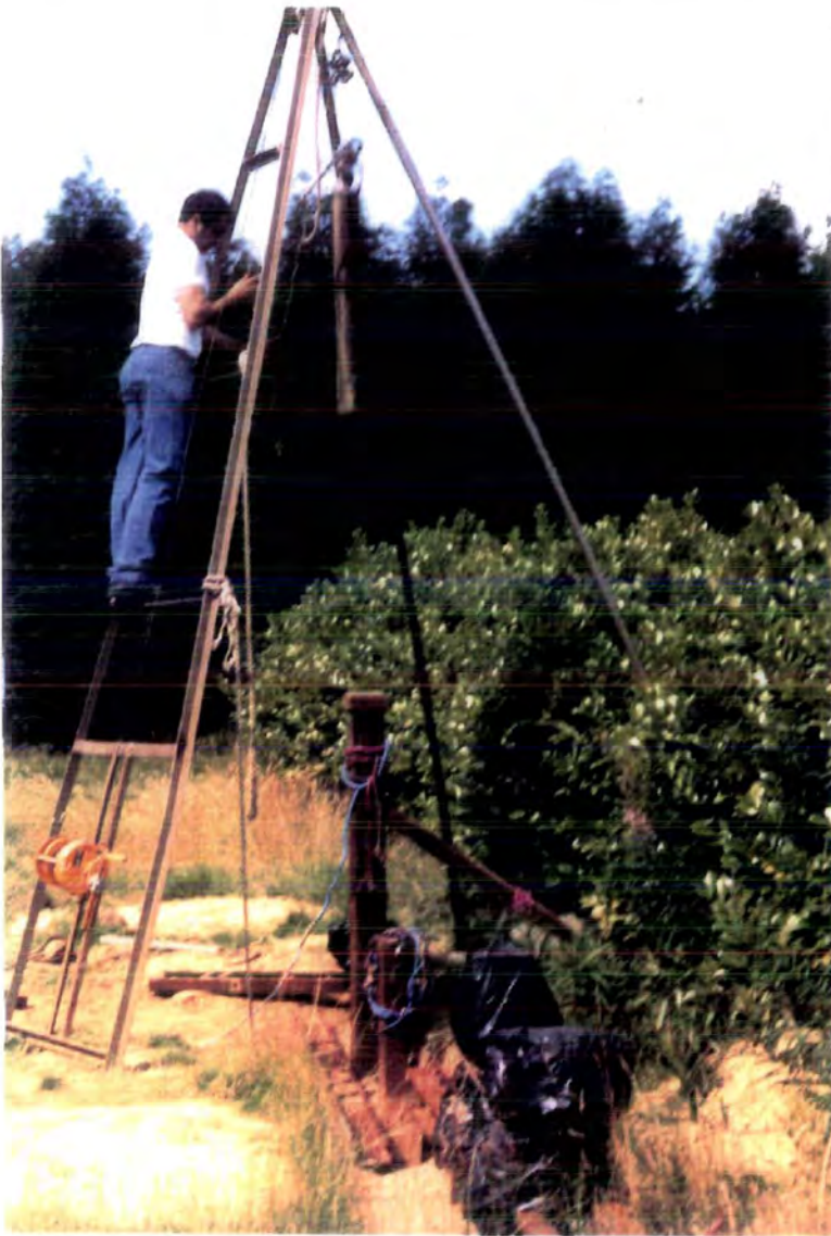
Plate 3.4 Pile driving technique.
