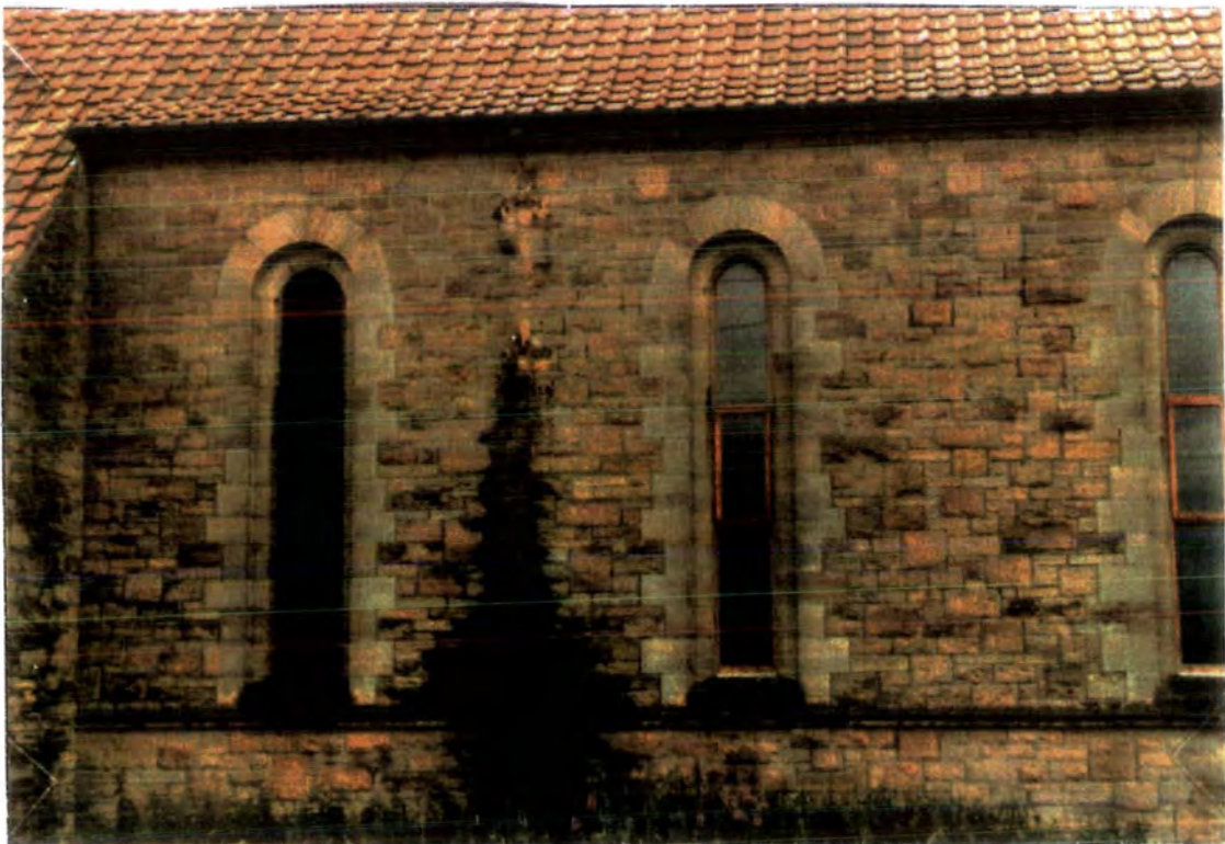
(20) The new hardwood windows (centre and right) do not quite fit in with their stone surroundings as did the one on the left (before it was barred)
