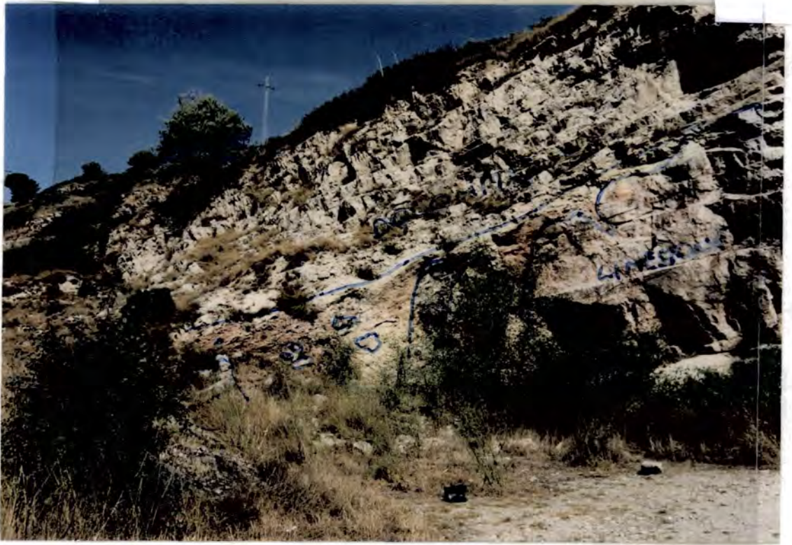
Fig. 4.25. Subsurface paleokarst at Centelles. Paleokarst deepens to the left of the view and is covered by orange-red marl containing blocks of dolomite and limestone. Karst separates dolomite above from limestone below. Centelles locality.
