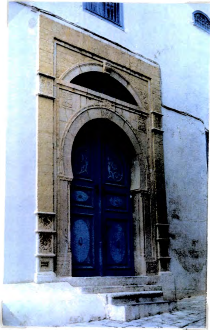
Plate 4: an elaborate entrance doorway, in this case that of Dar Cherif at Sidi Bou Said. Similar doorways are found all over the Medina.
