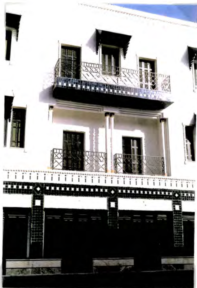
Plate 28: Bab Souika urban renewal area: apartment buildings on the Rue Bab Benat by T. Ben Miled and M. Ridane in a reworking of the style arabisant.
