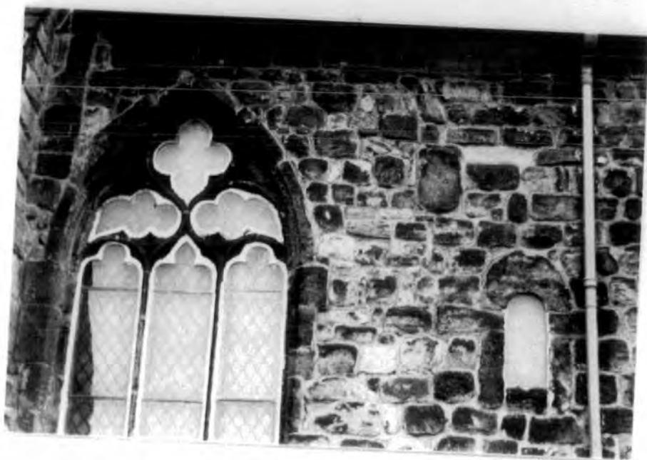
South wall exterior: upper doorway
