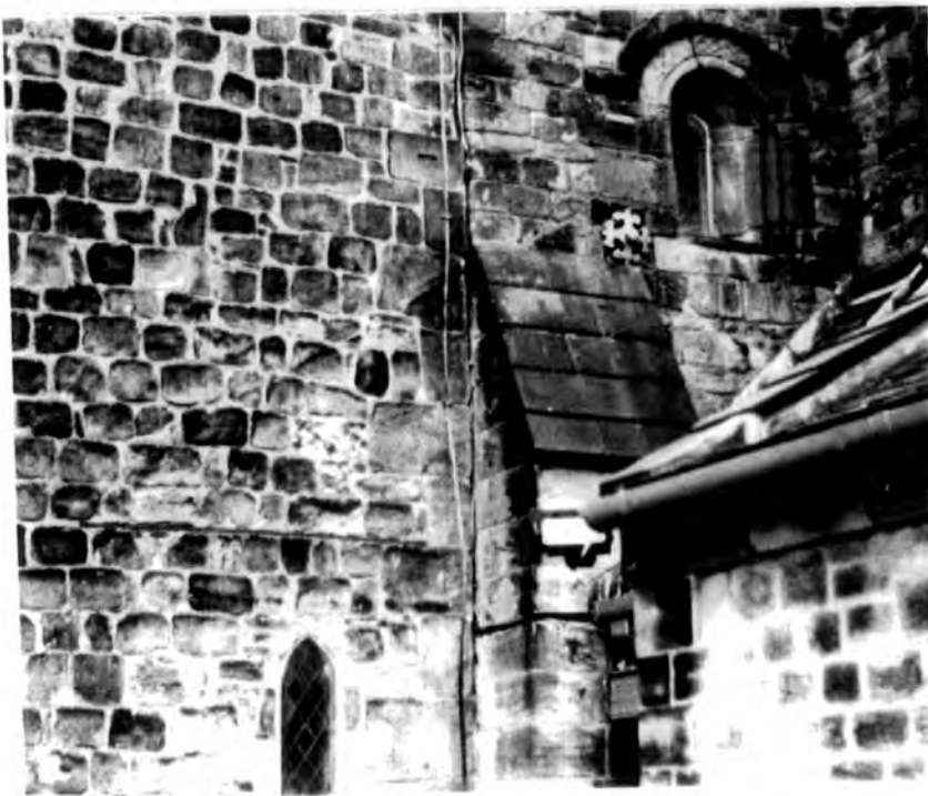
North wall: tower window and gable lines
