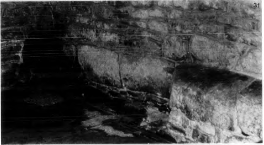
BRIGSTOCK South aisle stones and bench
