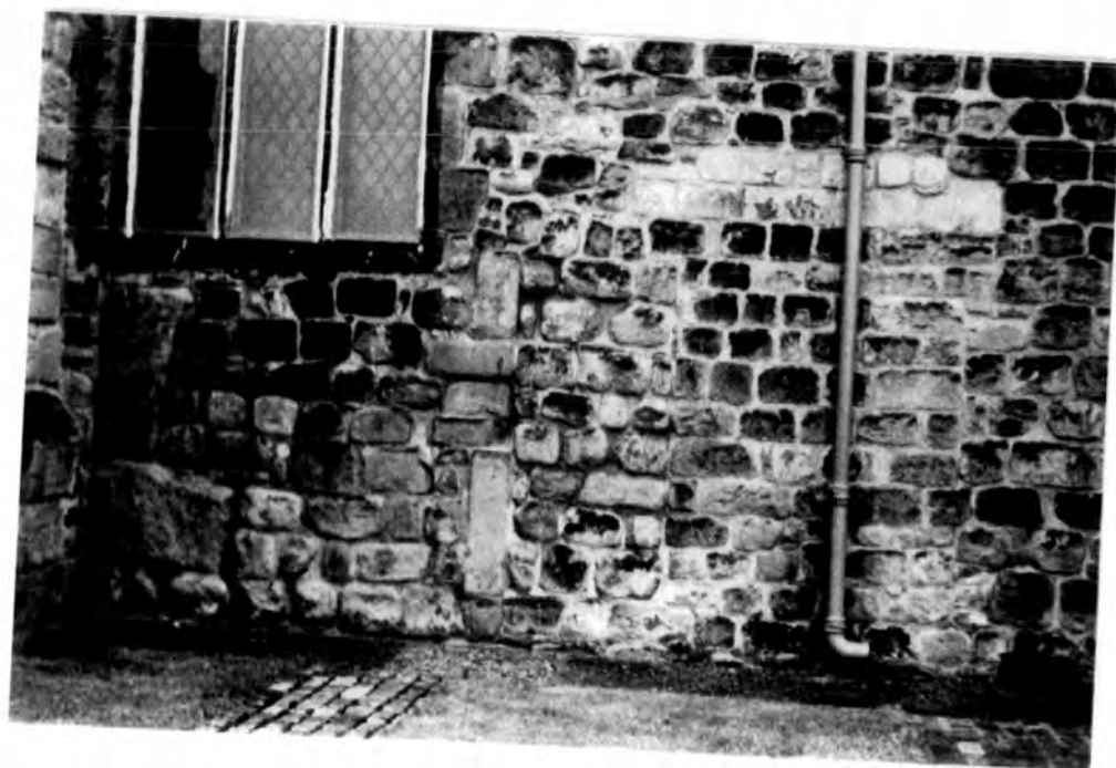
South wall exterior: lower doorways
