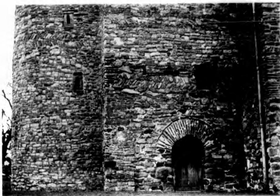
Lower tower and stair turret, south face
