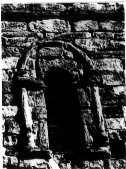
Detail: upper doorway on south
