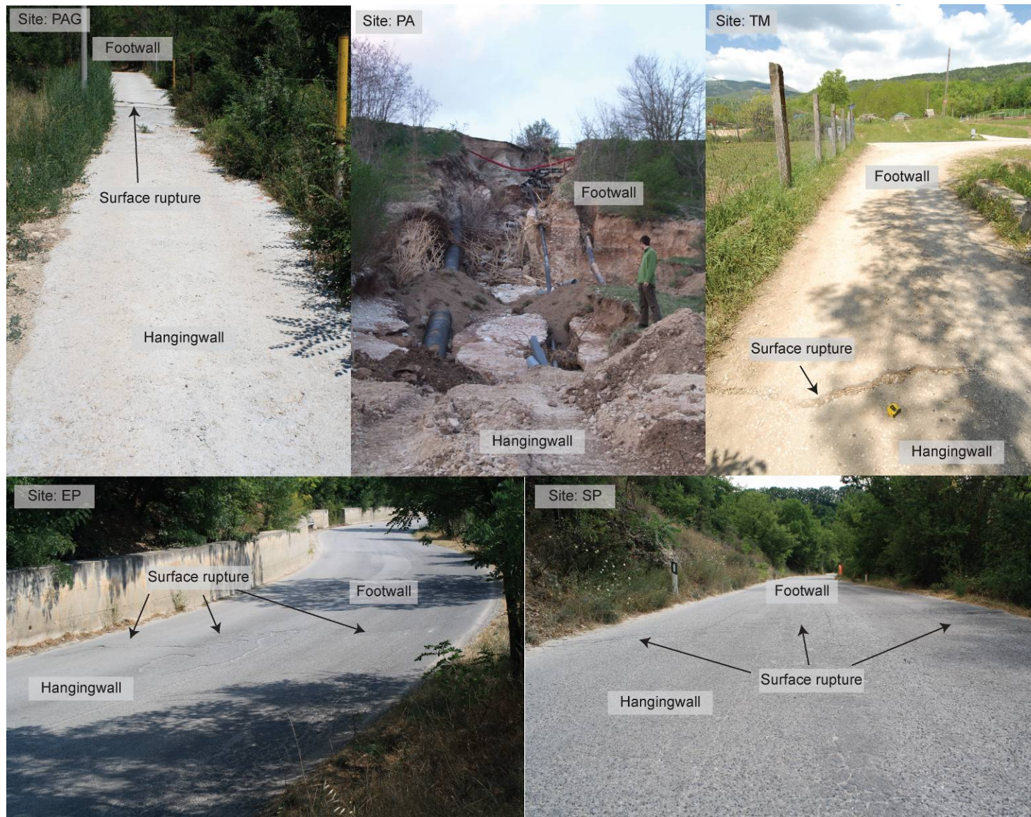
Figure 5.1.3: Field photos of the five L'Aquila earthquake surface rupture study sites where postseismic deformation was measured.
