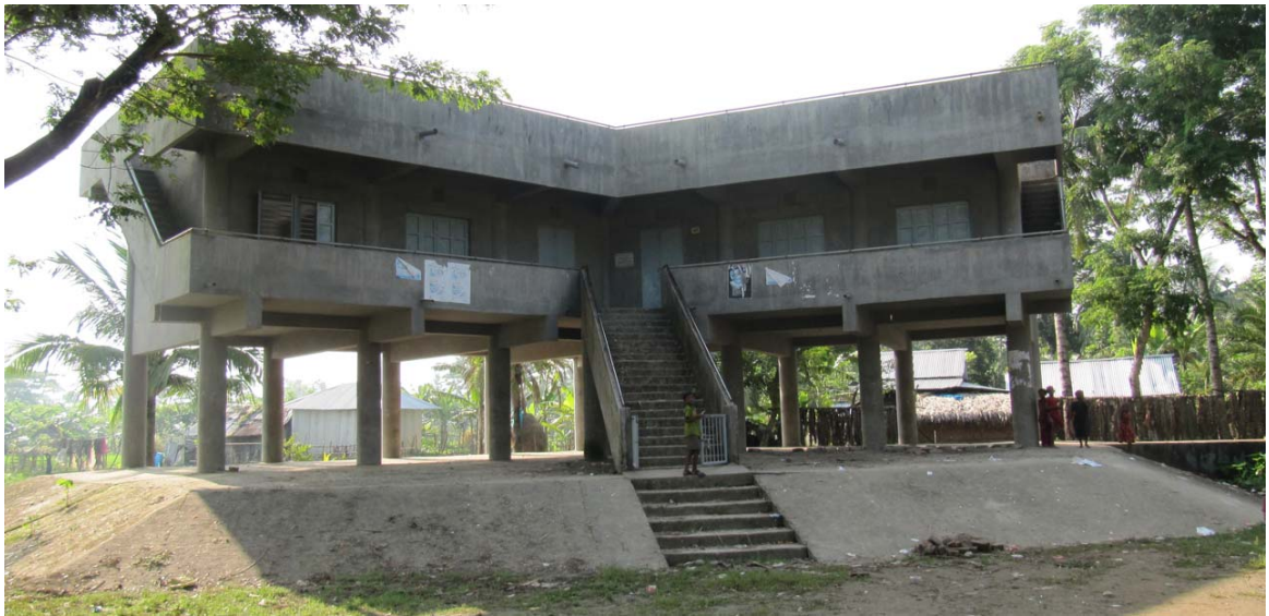
Figure 4.4: Gabtola Cyclone Shelter
