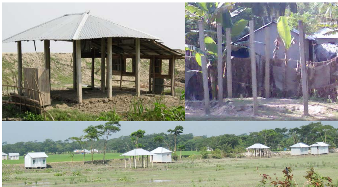
Figure 5.6: Abundance of abandoned houses – the construction cost (excluding material costs) for every single house was Taka 10,000, which make no sense now. All of the houses in a row in the bottom picture are now abandoned. (Source: Author)
