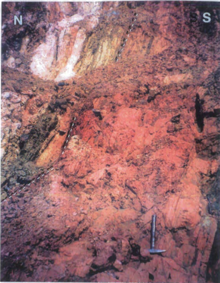
Photo 5.3.8- Concordant contact between siltstones and sandstones observed in the Serra do Sereno quartzite quarry.
