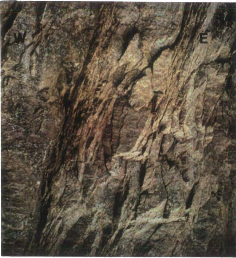
Photo 6.5- Set of N-S fractures concentrated in 30-50 cm zones separated by 1-2 cm of less fractured rocks.
