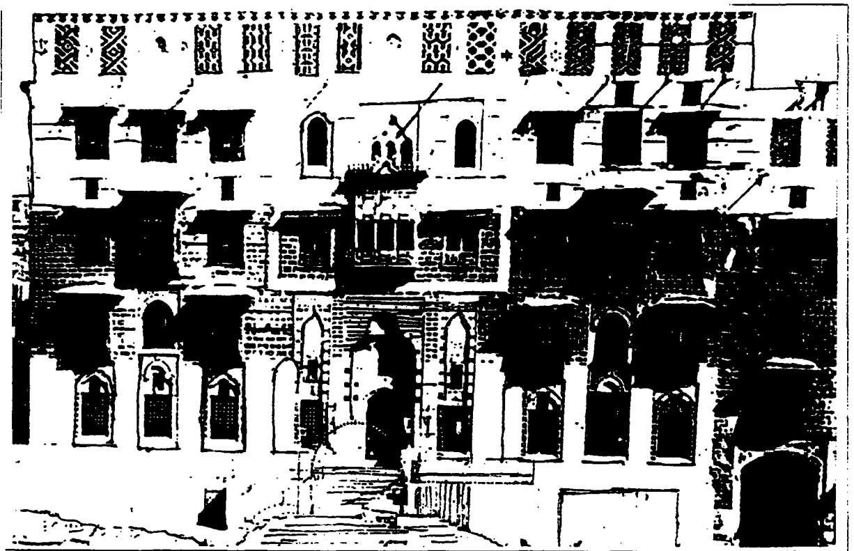
Fig. 3.11: House of the Sharif of Makkah, 1970 (Angawi, 1988, after a contemporary photograph)
