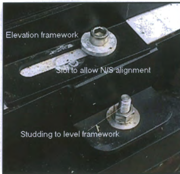
Photograph 2 Adjustment of elevation framework
