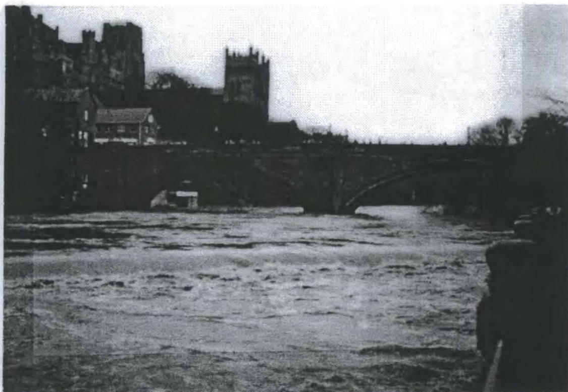
Fig. 1.6 Framwellgate Bridge, River Wear in flood (Durham Record 1991)
