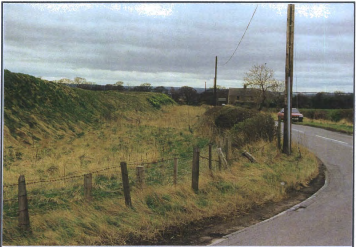
Fig. 5.16 Visual Impact Assessment. View from V4, looking south. Showing path section R12 - R13.
