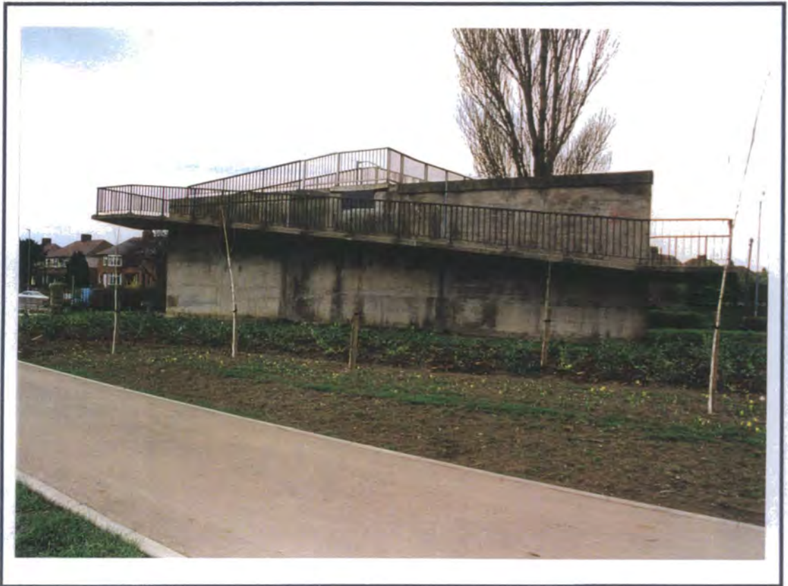
Fig. 5.11 Footbridge Crossing A167(T) Showing Restricted Visibility.
