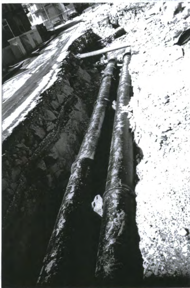
Plate 8.8. The Pembroke- Mosta pipeline being laid.
