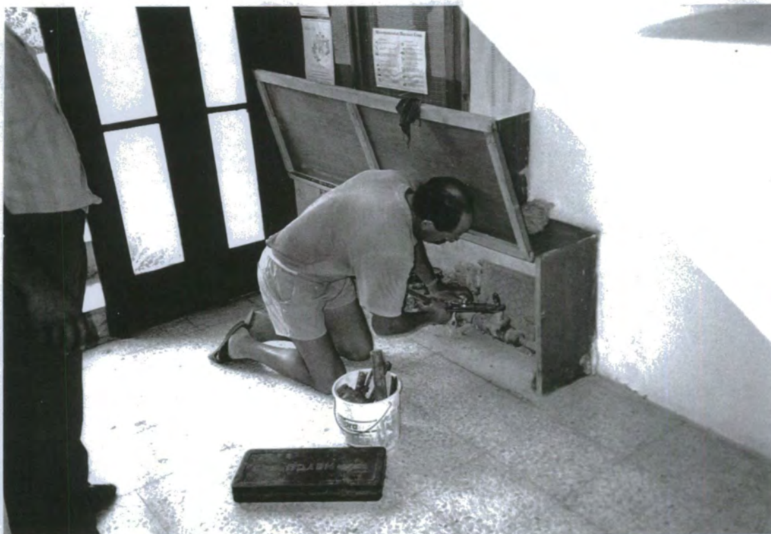
Plate 8.3. Meter replacement at the Sunny Isle Aparthotel (Msida).
