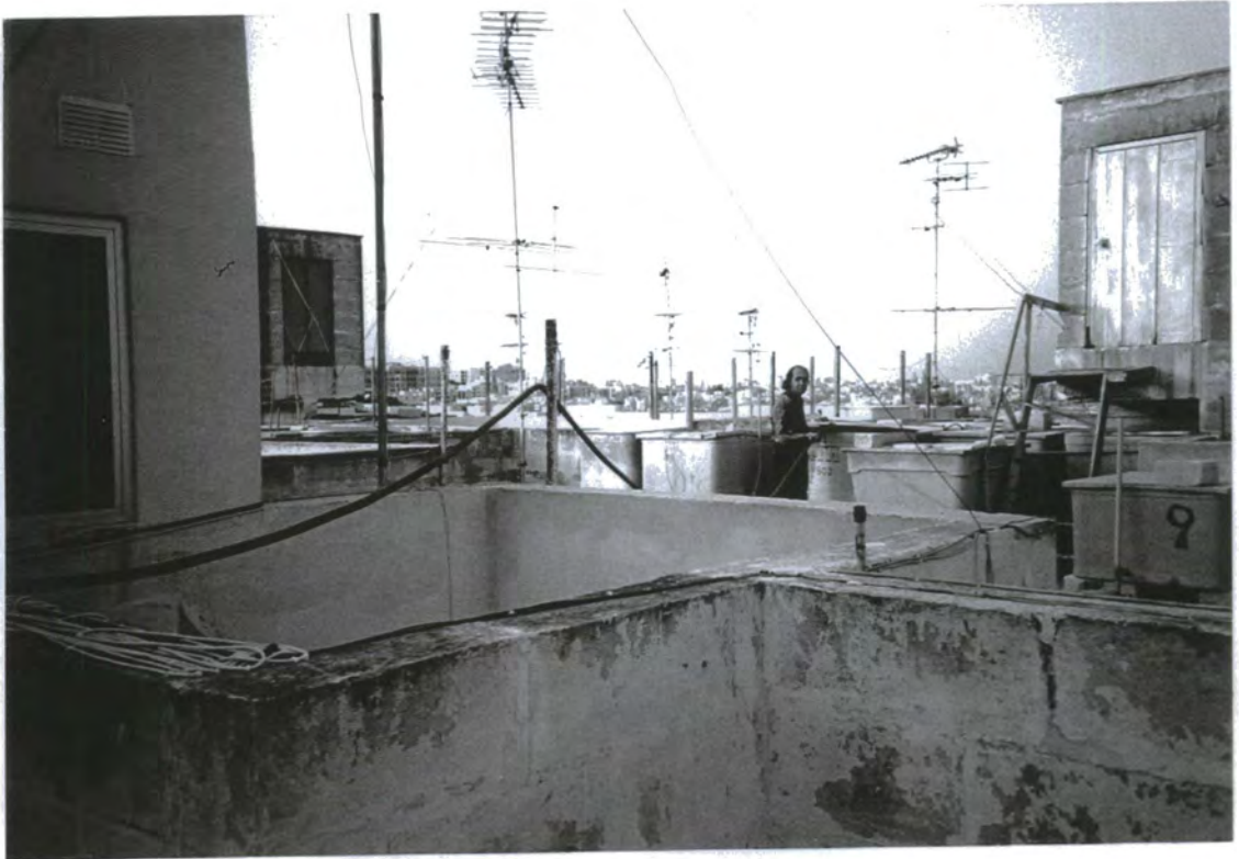
Plate 6.2. Water tanks on rooftops.
