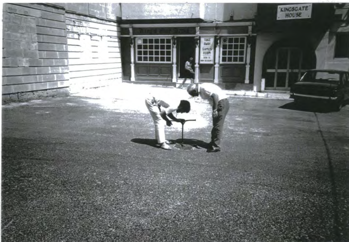
Plate 8.7. Daytime leakage detection.
