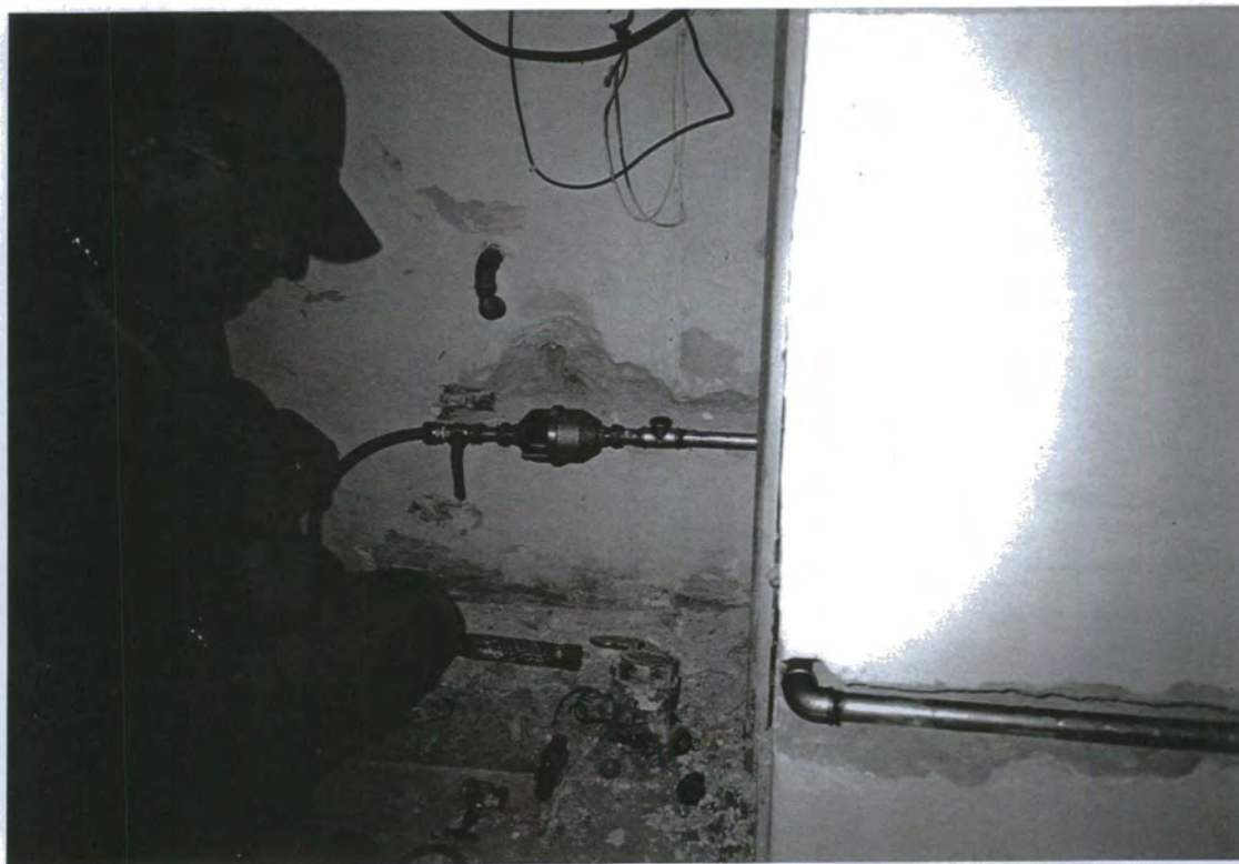
Plate 8.6. The new class 'D' meter being installed.
