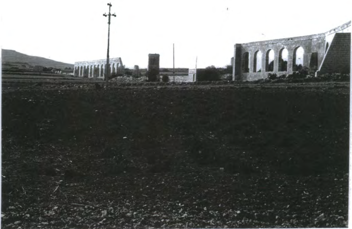
Plate 2.8. The ruins of the aqueduct in Gozo.
