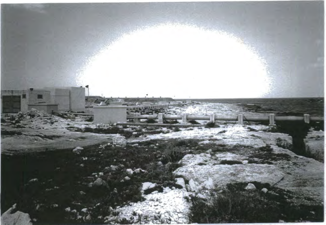
Plate 3.4. The feedwater inlet and brine reject pipes at the Pembroke RO plant.
