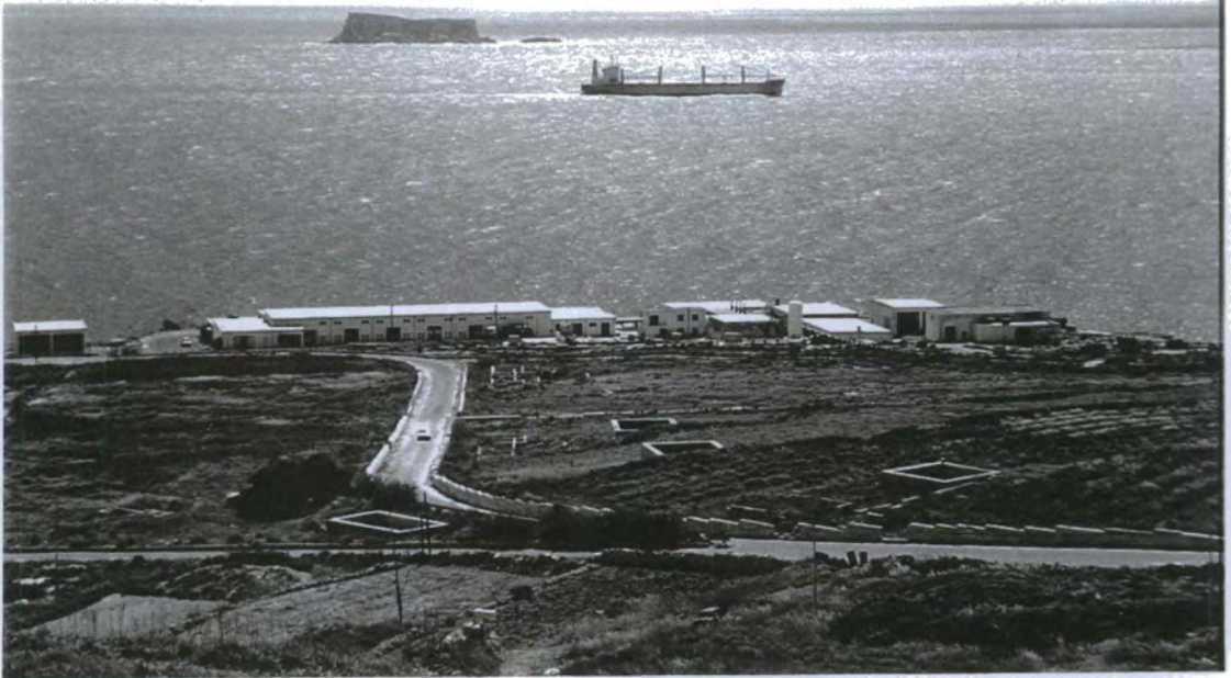
Plate 5.1. Sea traffic passing close to the Ghar Lapsi RO plant.
