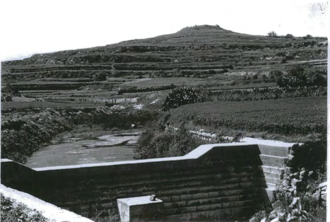
Plate 3.19. Surface ponding behind a dam in a wied .
