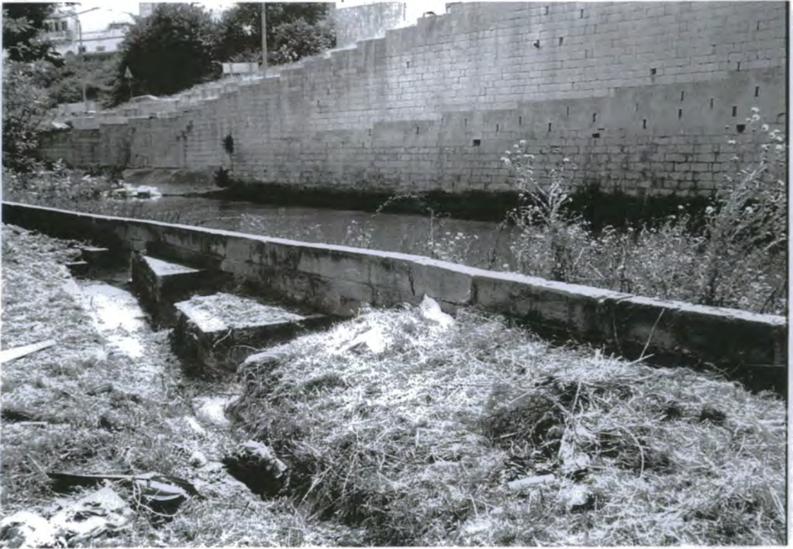
Plate 3.1. A disused open reservoir in Msida.
