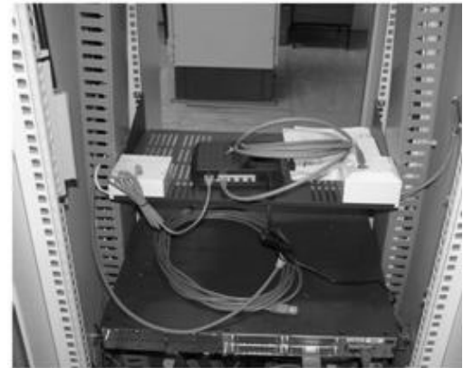
Figure 55: Substation relay: a) input from meteorological station (Figure 1). b) modem for communication to the outside world
