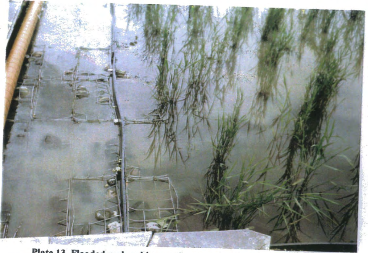
Plate 13. Flooded rock-gabions and pot-grown Phragmites australis inlet section of the CATS Terminal reedbed, 14.00 hours, 1/7/97.
