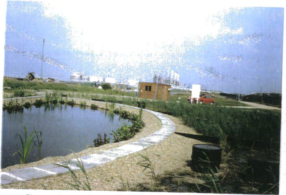
Plate 17. Pot-grown Phragmites australis section of the CATS Terminal reedbed, July 1997, showing a decrease in shoot-density away from the inlet section. (Local reed inlet section in the foreground showing less successful establishment of planted reeds)
