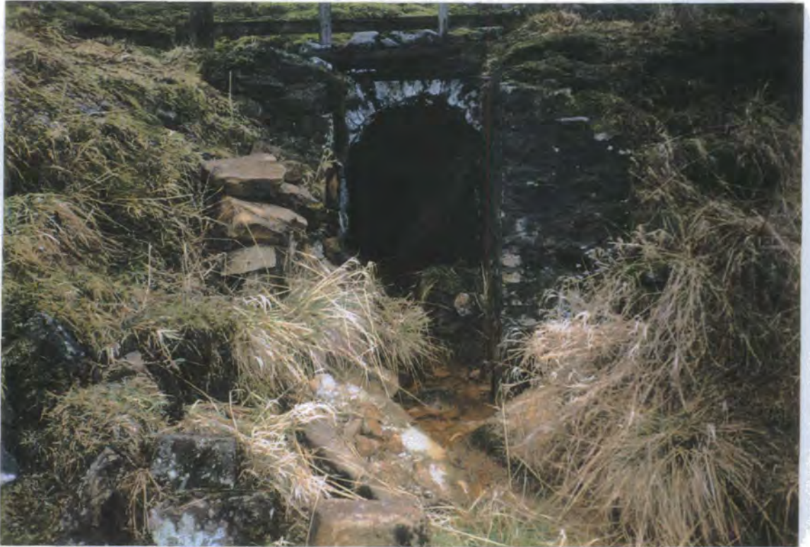
Figure 17.4 Drift Entrance - Iron
