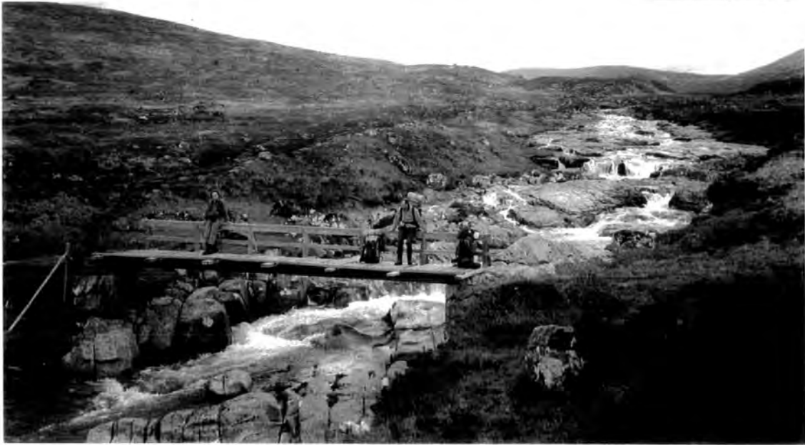
Figure 6.7 Footbridge over Uisge Labhiar, Inverness-shire, Scotland
