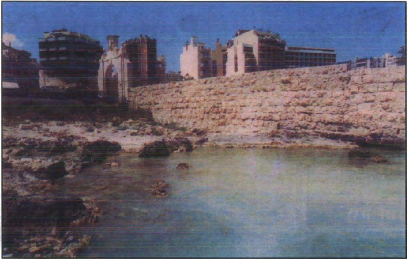
Plate 7.2 Malta: St. Julian's Bay: problems of dilapidation in urban areas spill over to the near shore waters with sewage and liquid overflows in bathing zones. Source: The Times 14 th August 2001
