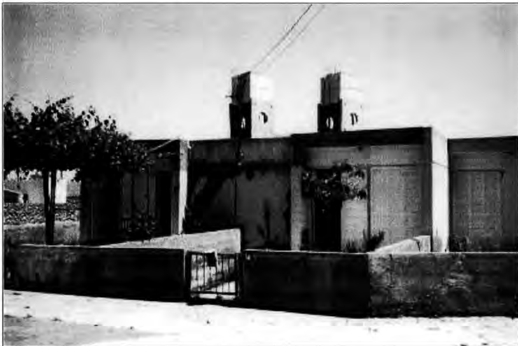
Houses were often constructed rapidly, to poor standards. Maintenance problems and ambivalent feelings toward houses can leave them looking very poor.
