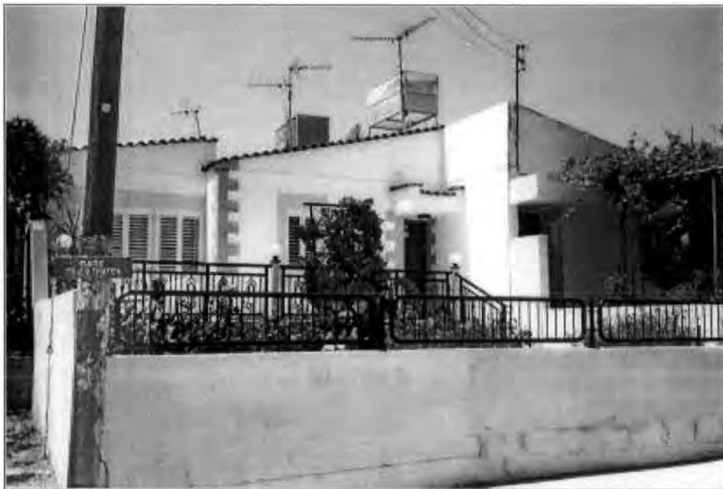
Ownership of title deeds enables refugees to use their property as capital for loans that can be used to alter the appearance of the house. The identity of the house on the left has been dramatically changed to suit Cypriot aesthetic notions of design. It contrasts with the house on the right, which retains the monotonous and industrial appearance of social housing.
