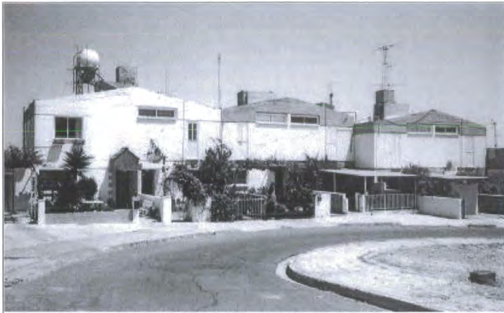
The house on the left of this picture, has recently undergone investment after the owner received title for his property. New windows, an extension (on the far left) and a new roof-mounted heating system have all been added. Other houses retain the appearance they had when they were first constructed.
