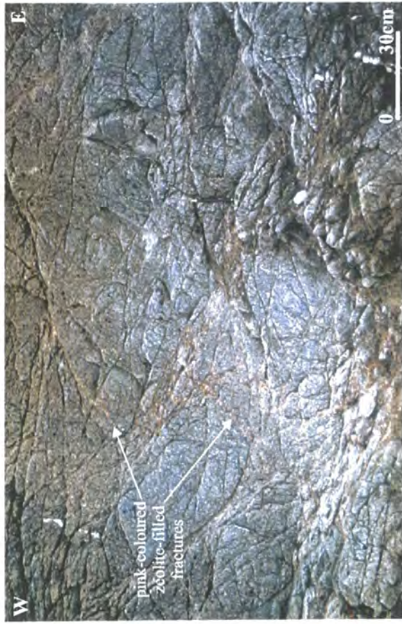
Figure 6.18 Zeolite-filled fractures observed adjacent to the AVFP at locality SA 7.
