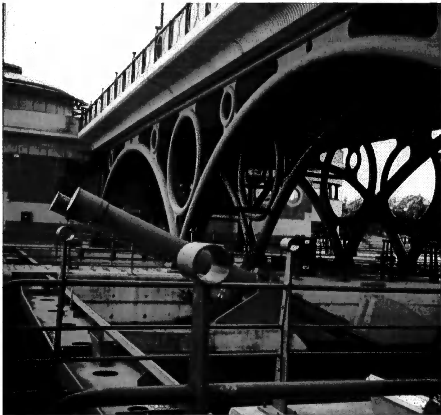
Figure 1.3. The hydraulically controlled flap-gates of the Tees Barrage.
