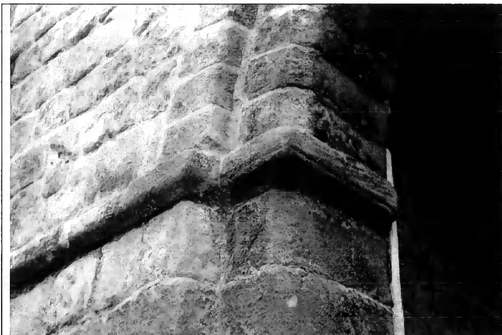
Plate 21 A Detail of the Impost and Arch of the Outer Face of the Gatehouse at Prudhoe Castle
