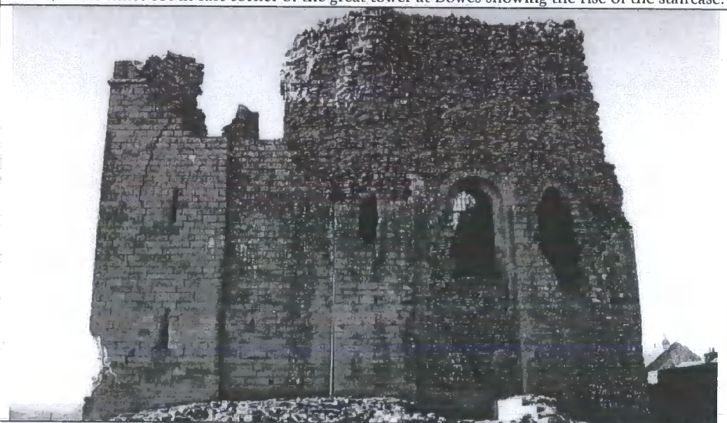
Plate 72 The east face of the great tower at Bowes
