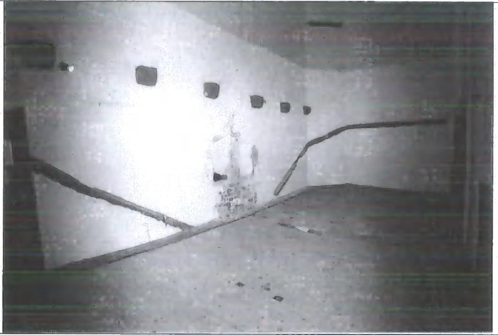
Plate 61 The twelfth-century roofline at Appleby.
