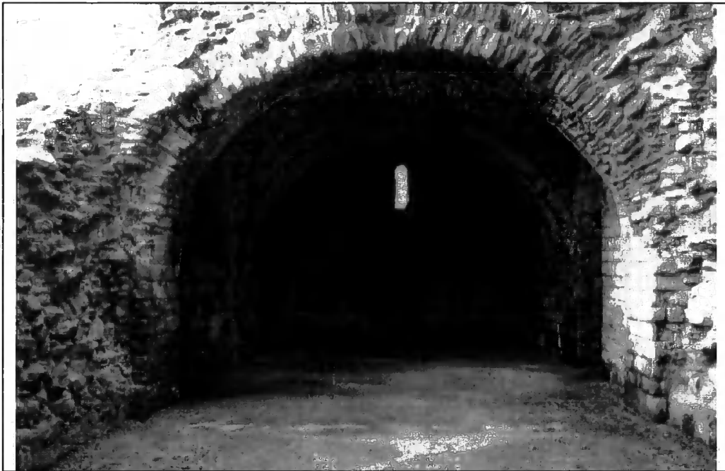
Plate 19 The Cellar of the Phase I Keep at Norham Castle
