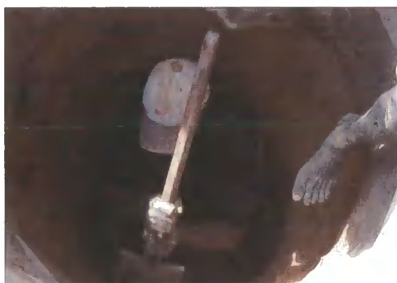
Figure 6.6 Digging the latrine to 3.5 metres
