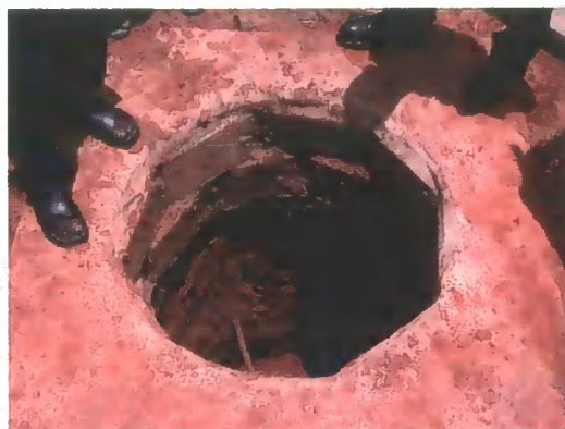
Figure 6.5 Completed latrine 'collar' ready for digging
