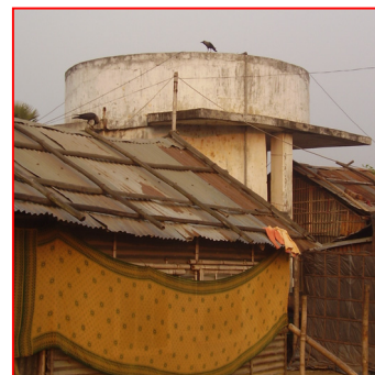
Figure 6.6: Overhead water storage tank in BT
