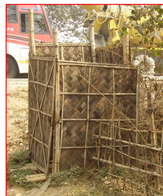
Figure 6.11: A handmade latrine with locally available materials
