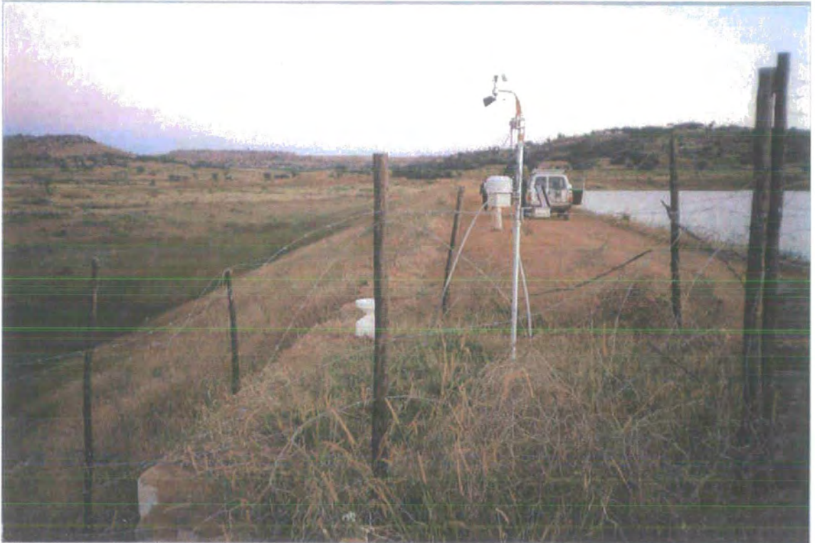
Plate 2.1. An automatic weather station on the dam embankment.
