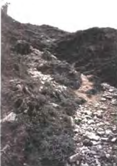
Plate 2.3: The condition of the trail to the roadhead after the monsoon
